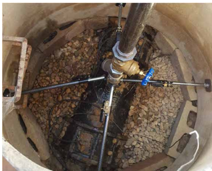
Figure 9 – Hydraulic Transient Induction Point (Transient Generator Station)
