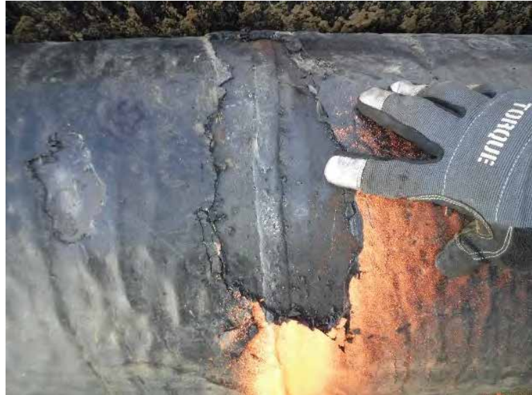
Figure 5 & 6 – Outer Coating Removal to Check Bonding (orange color is from paint)
