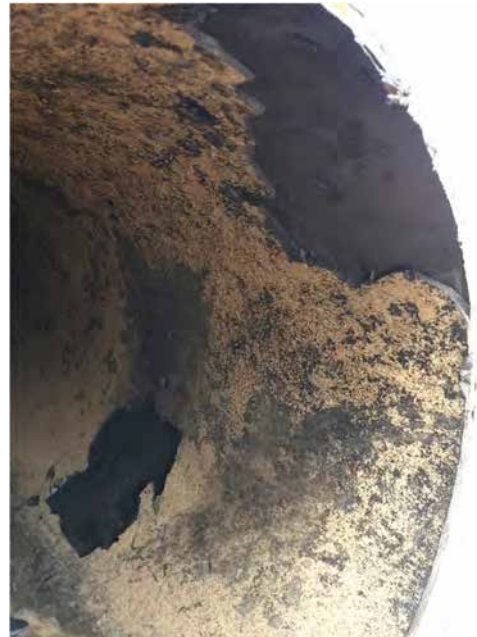
Figure 8 – Interior Coating Removal to Check Bonding
