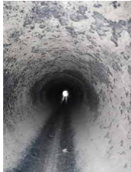
Figure 7 – Interior of Pipeline
