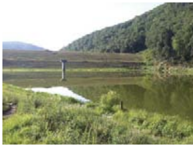
FIGURE 1: Hone Quarry Dam in Rockingham County
