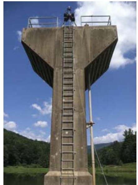
FIGURE 3: Hoisting inspection equipment onto riser structure
